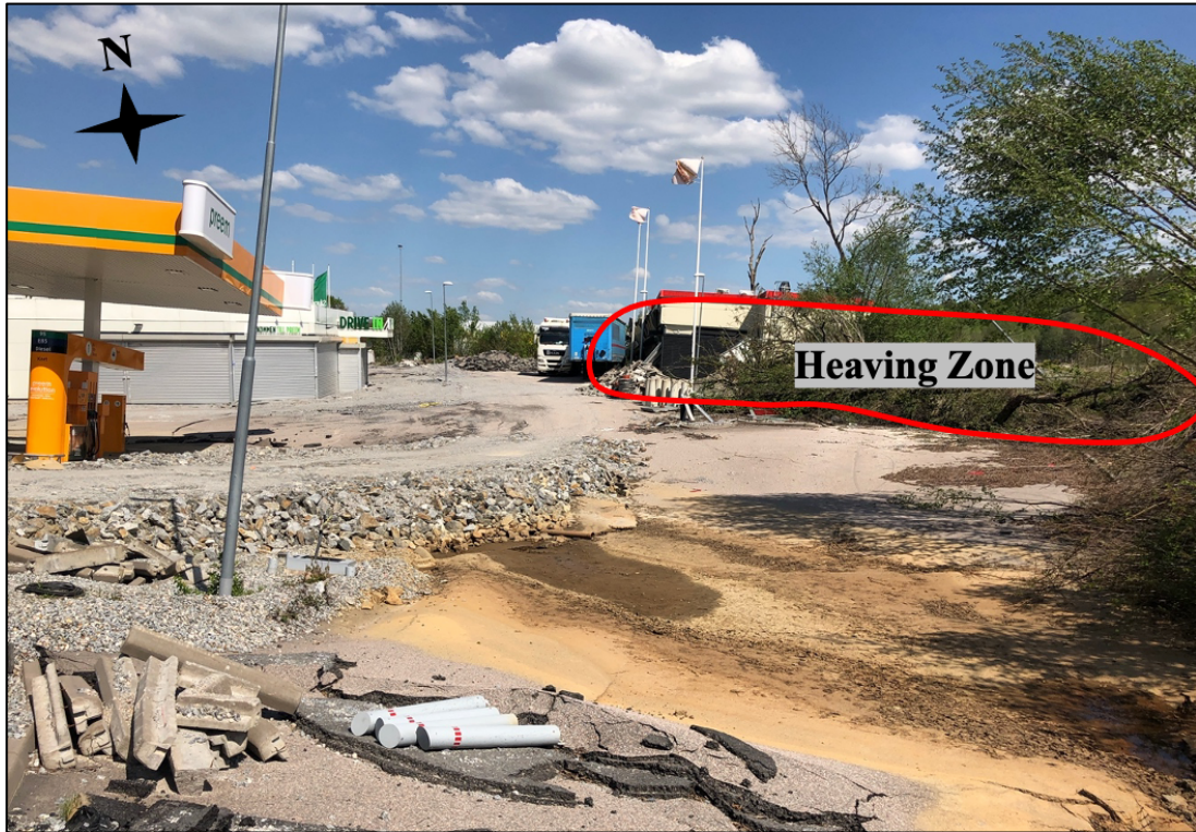
Figure 20 Photograph taken in the northwestern part of the landslide. This shows the impact that the landslide had on buildings and infrastructure. One of the heaving zones are also part of the image.
