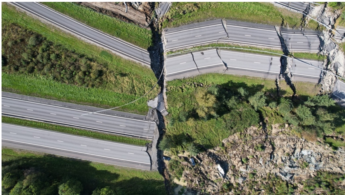
Figure 1 An UAV-image showing how the landslides has dislocated the highway E6 from its original place (Länsstyrelsen, n.d).
