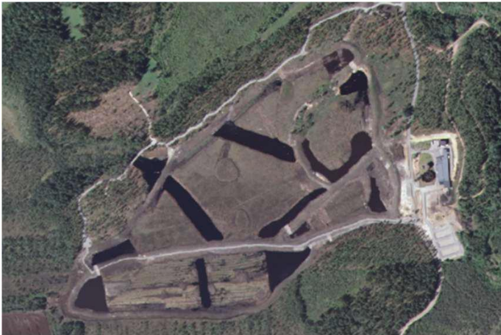
Figure 2. Aerial image of the ponds during construction, showing the deeper sections (Kullingsjö, 2025).
