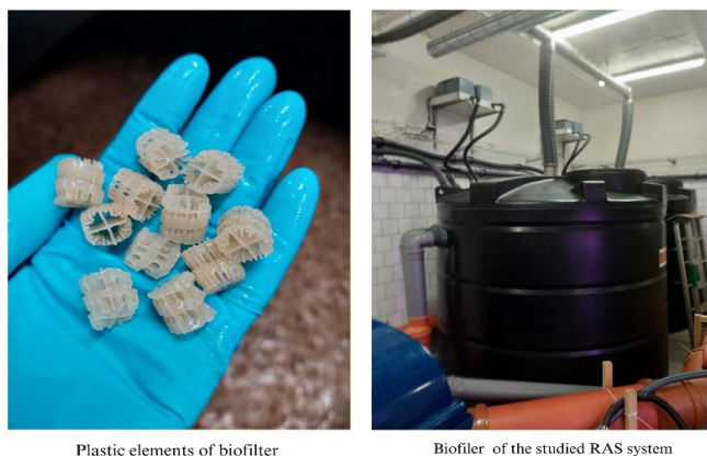
Figure 3: Plastic carries of the biofilters and biofilter of the RAS
