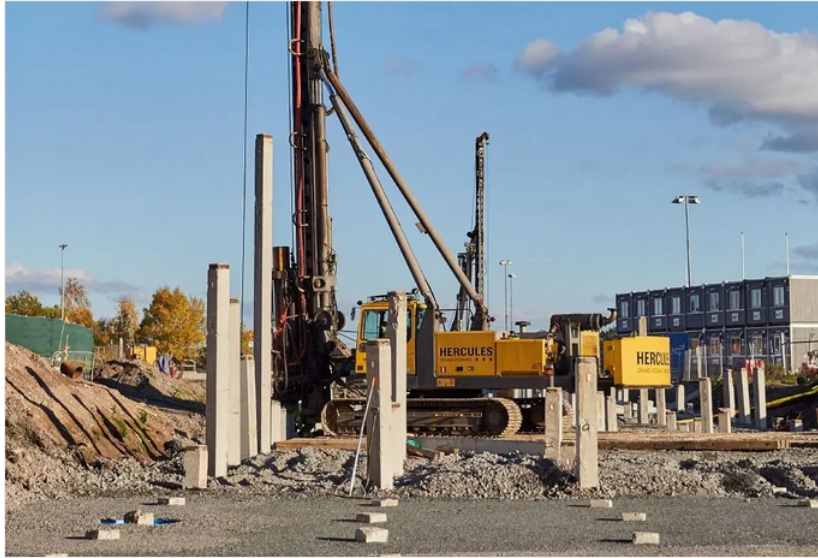
Figure 2: Concrete piles at installation [1].
