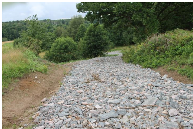
Figure 19: The picture is from 2023 with several layers of crushed gravel/macadam.
