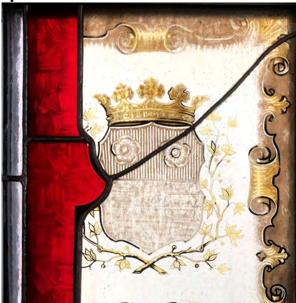
Figure 21. A panel of the red window in the church's choir with paint loss in the dark trace lines. Photo: Eisfeldt, 2022
