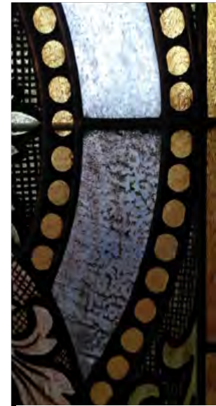
Figure 60. Photo of the dirt of the left window of the Linnea church. Photo: Eisfeldt, 2022
