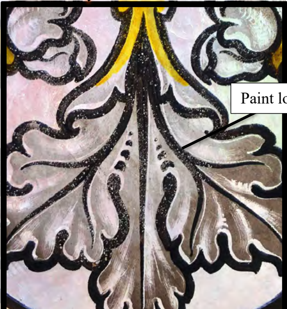
Figure 42. Example of loss in form pin-holes found on the rose windows. Photo: Eisfeldt, 2022
