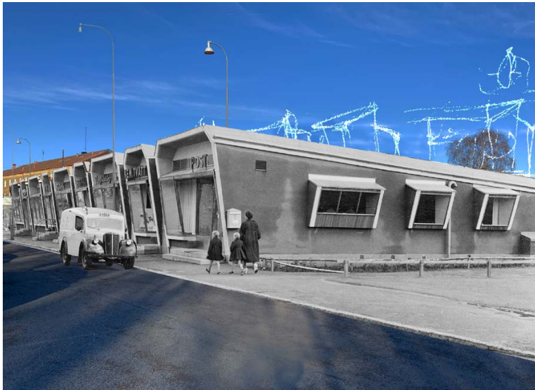
Figure 43. Horizontal from the stores and vertical aspect from the punkthusen in the back
