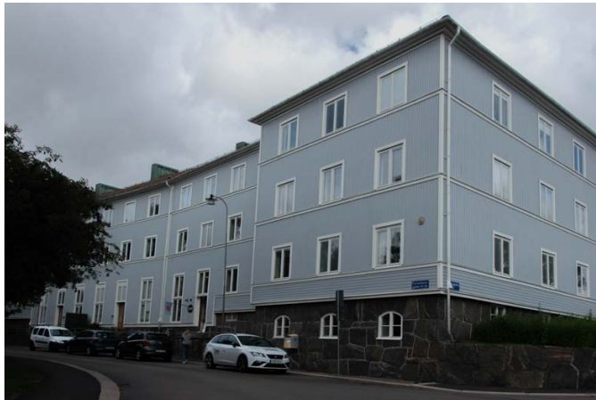
Figure 5. example of a landshövdingehus from HSB, Gothenburg
