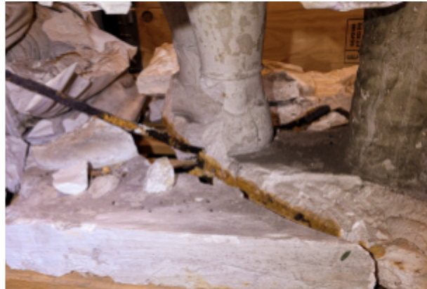
Fig. 7 - Deformed armature protruding from one of the sculpture's feet. Break edges are clearly visible where the plaster has fractured as a result of corrosion. Stockholm Stadsmuseum. SSM 31130.
