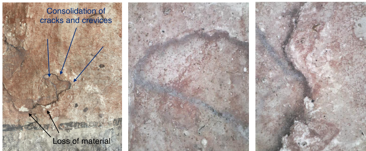
Figure 57 (left): Area R1: after 1st application with Nanorestore ®
