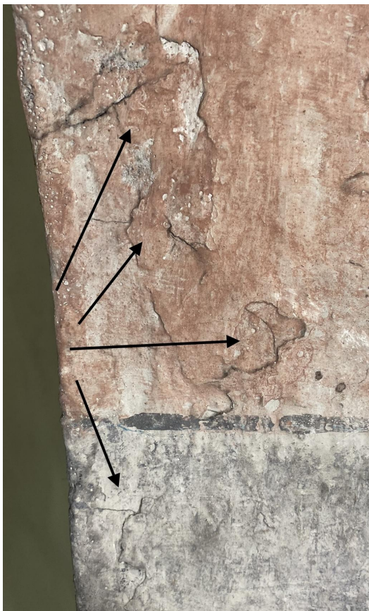
Figure 2 (left): Loss of adhesion between paint layer and substrate (flaking of painted layer) in block painting in belt arch
