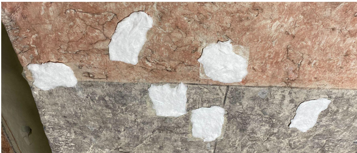
Figure 21: Application of nano-lime products with Japanese paper and cotton compresses
