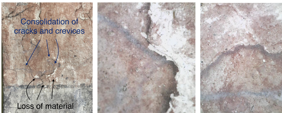
Figure 69 (left): Area R1: after 2nd application with Nanorestore®
