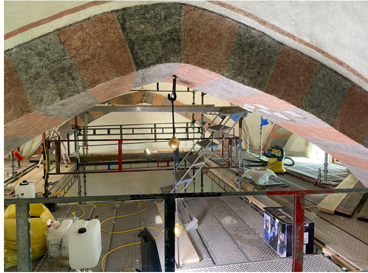
Figure 6 (right): Pointed belt arch
