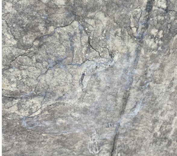
Figure 53 (right): Area B2: After treatment with Nanorestore Plus® and retouching 6
