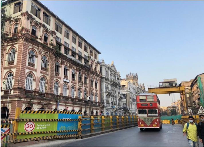
Figure 29: Metro construction on DN Road
