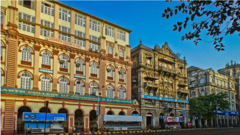
Figure 12: Street view of DN Road
