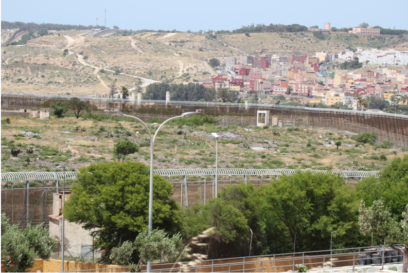
Image (39): Installed 'peines invertidos'. Photograph taken by the author in May 2022.
