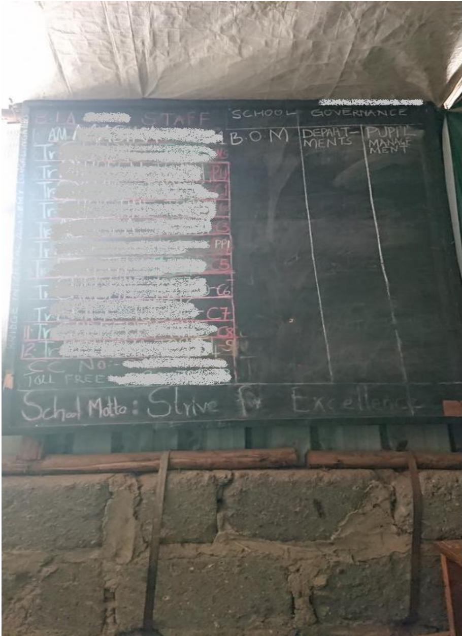
Figure 5.13: Photo from a BIA office. Blackboard displaying teacher names and responsibilities, hanging on a wall made of brick and mortar, sticks and corrugated iron. The roof was also made out of corrugated iron sheets, and the fabric is likely hung underneath it to give some protection against the heat, and perhaps to counteract sound levels a little. (Photo: Author's own.)
