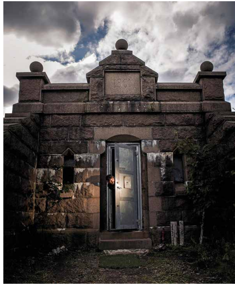
Figure 42. Musician Jorge Alcaide at the metal entrance door of what used to be the Gråberget water reservoir and has now become the Kulturtemplet (the Culture Temple). Picture by Nicke Johansson, published in Göteborgs Posten 'Så ser livet ut inuti Göteborgs vattentorn', 16 October 2021
