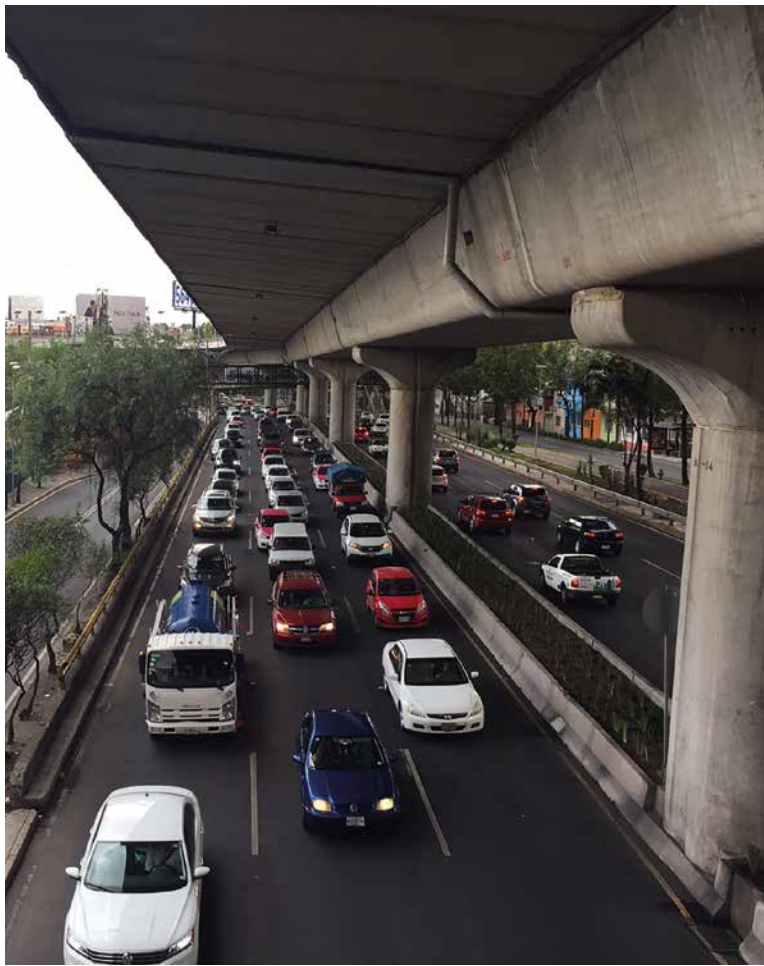
Figure 24. Peripheral ring road Anillo Periférico, as seen towards the north from the pedestrian bridge at its intersection with Avenida Constituyentes. Mexico City, June 2017.
