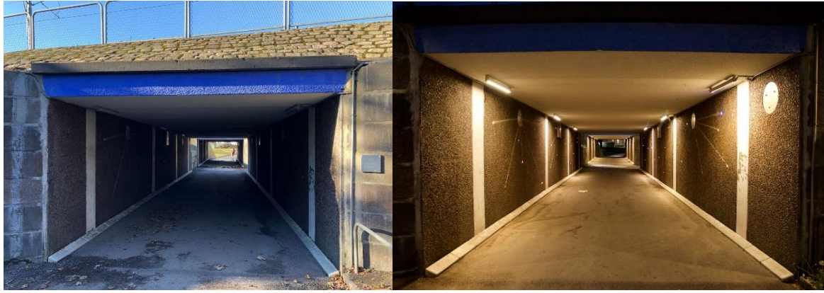
Image 5: Tunnel at Briljantgatan, daytime and nighttime. Photo: Louise Ringeby
