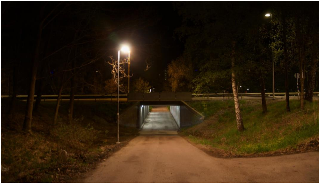
Image 7: Tunnel below Yrvädersgatan and connecting to Blidvädersgatan in Biskopsgården, by night. Photo: Louise Ringeby
