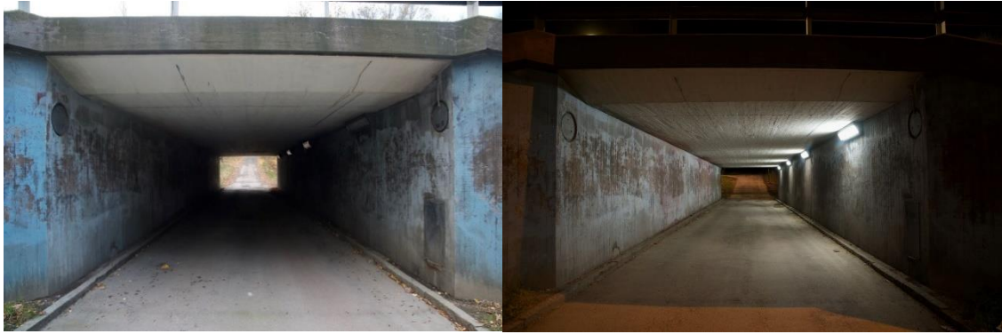
Image 2: Tunnel below Yrvädersgatan, daytime and nighttime. Photo: Louise Ringeby
