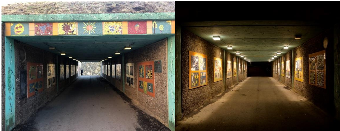
Image 3: Tunnel at Södra Fjädermolsngatan, daytime and nighttime. Photo: Louise Ringeby
