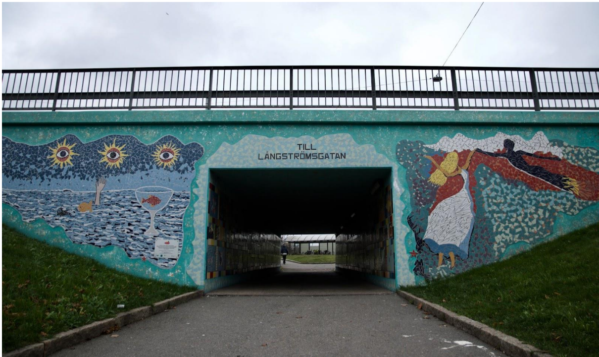
Image 1: Tunnel with mosaic art at Ekeströmgatan tram stop. Photo: Louise Ringeby.
