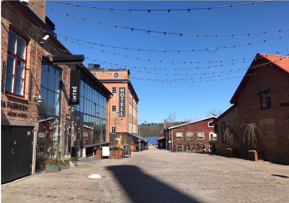
Figure 24. Nääs Fabriker contains several buildings all related to the earlier textile production.
