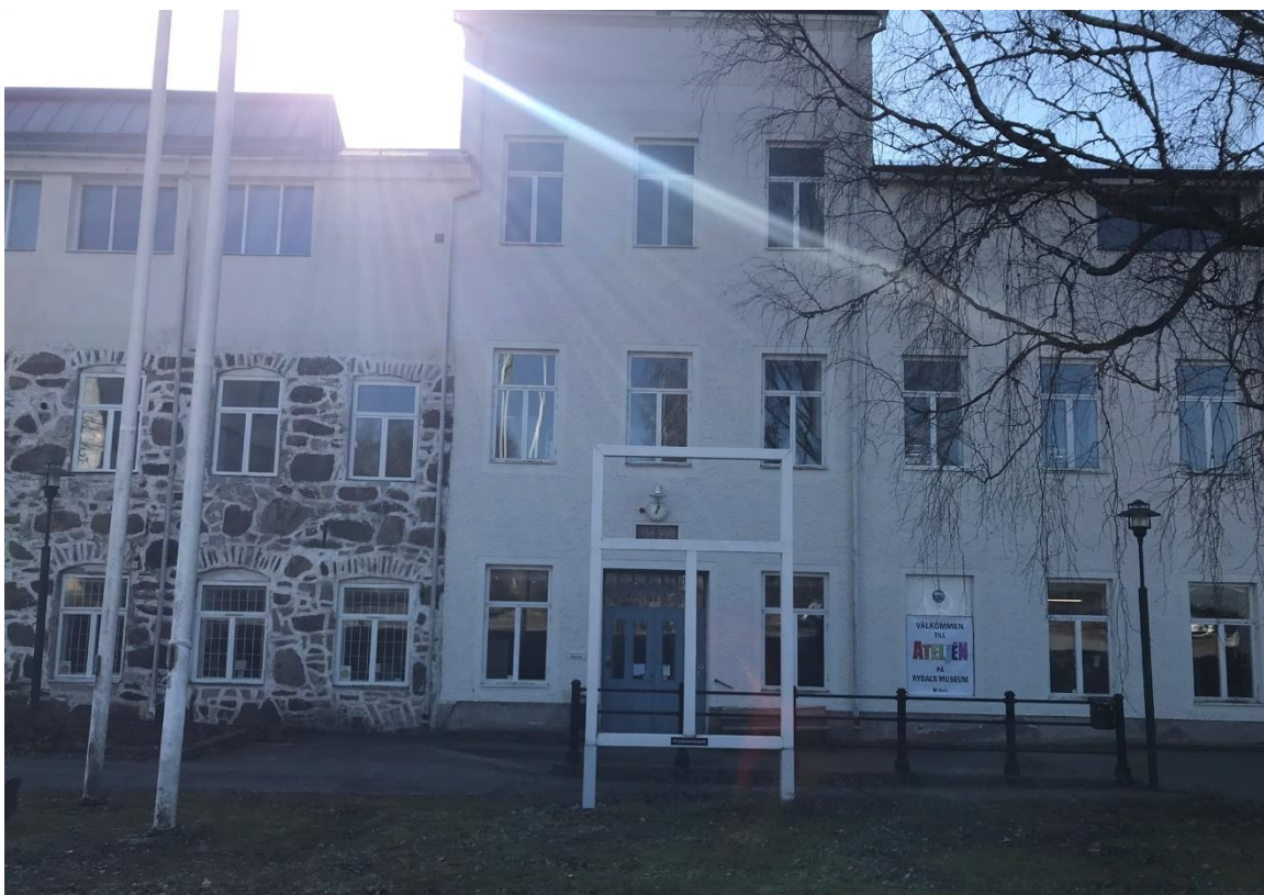
Figure 17. The northeast façade of the old spinning mill.
