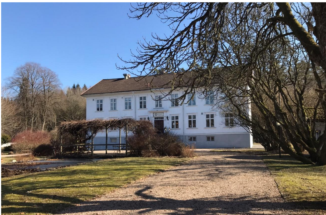
Figure 20. The managing director's house, today a restaurant.
