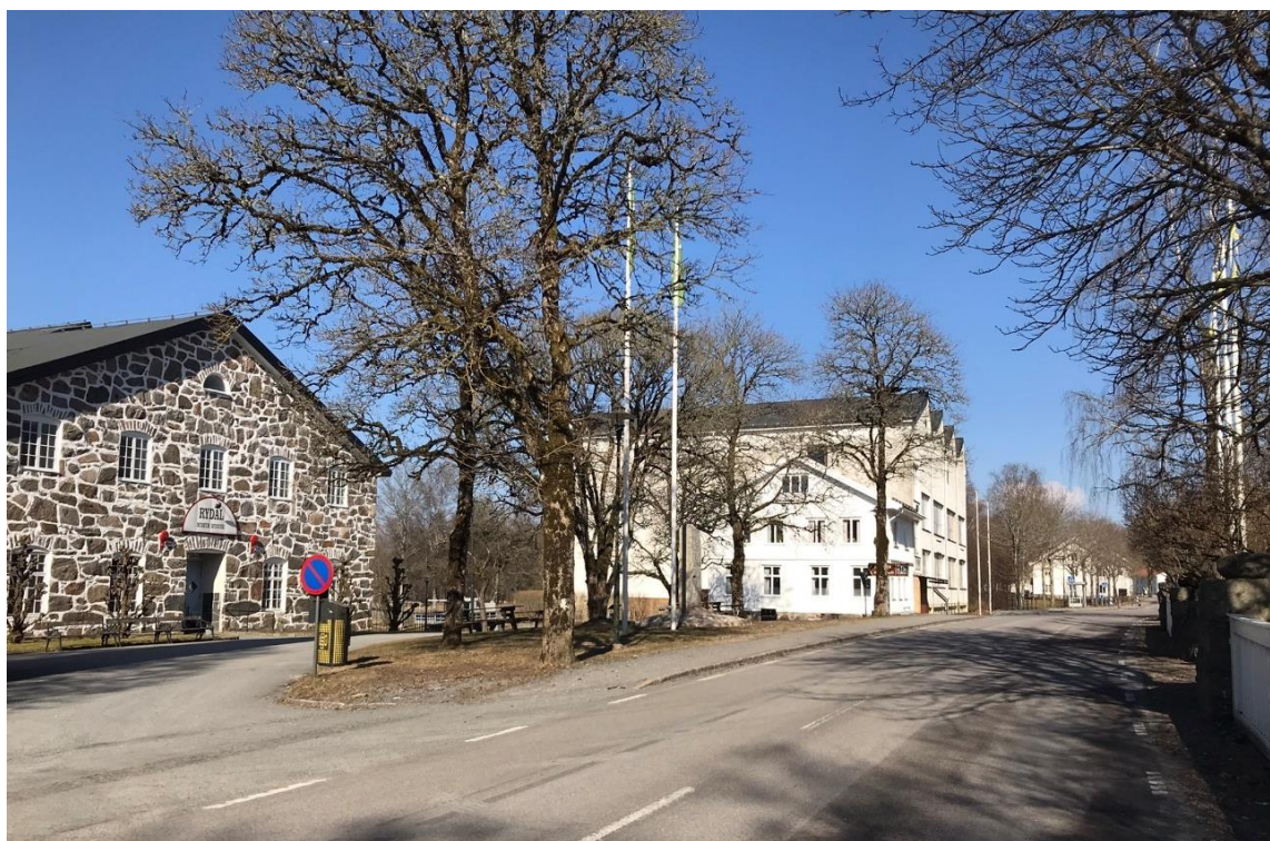
Figure 19. The old spinning mill to the right and the ‘new’ factory in front.
