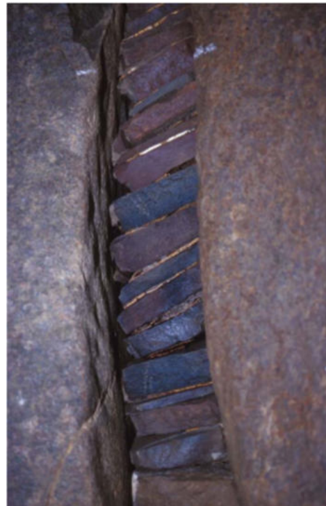
Fig 16. Birch bark between the stone slabs in the drywalling (Dehn 2012).
