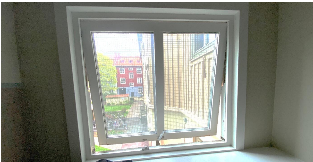
Figure 16. Projecting top-hung single-light window with 'false' central bar, seen from stairwell.
