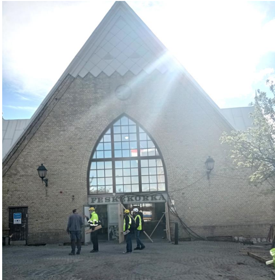
Figure 30. Arfvidsson, Bjelke-Holtermann, Mattson and a timber craftsman outside the west façade.
