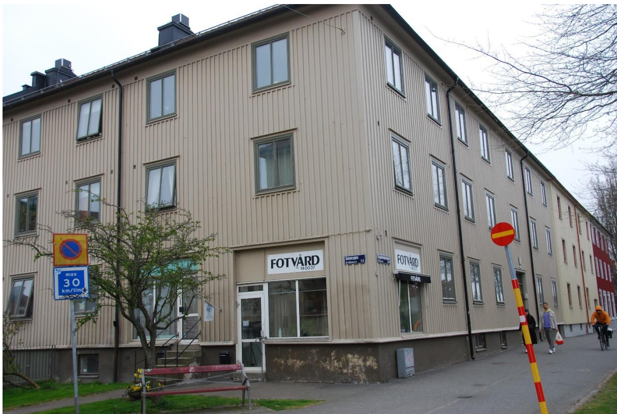
Figure 11. North-west corner of governor's house.
