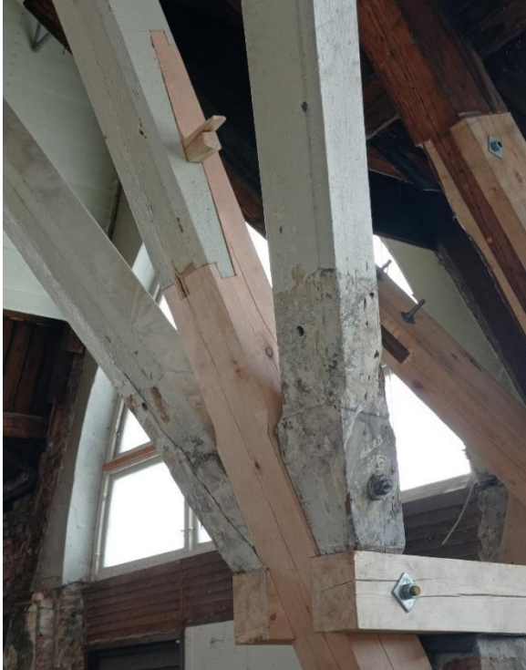
Figure 27. Repair on visible part of structure.
