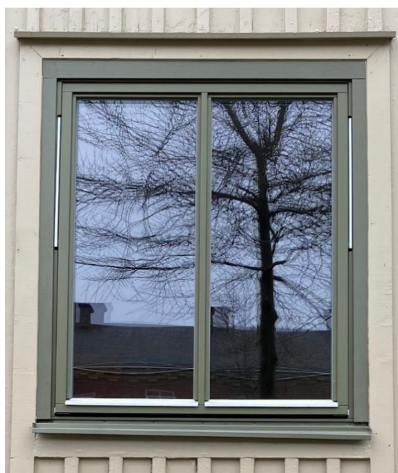
Figure 17. Close-up of window exterior.
