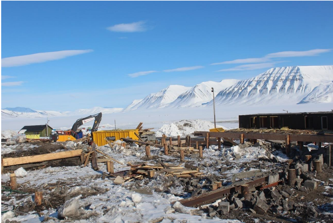
Figure 3: Demolition carried out by Decom. Photo: Kaisa Nordlund (2021)
