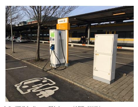
Figure A.2: CDC feeding an EV charger (ABB, 2019b)
