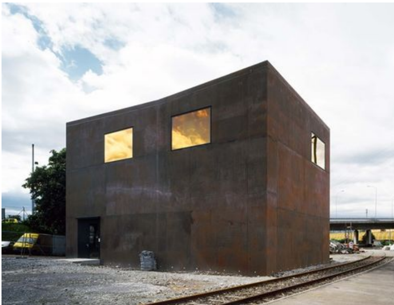
Fig. 25. The picture of the railway switching station shows the colour connection between the facades and the rusty of the tracks. Stellwerk Vorbahnhof , by Annette Gigon and Mike Guyer, 1999.
