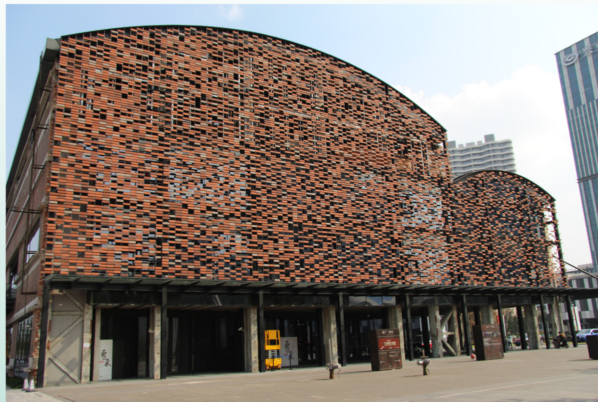
Fasad »exterior curtain», Shipyard 1862 i Shanghai, Kengo Kuma and Associates. Foto: Kristina Fridh.
