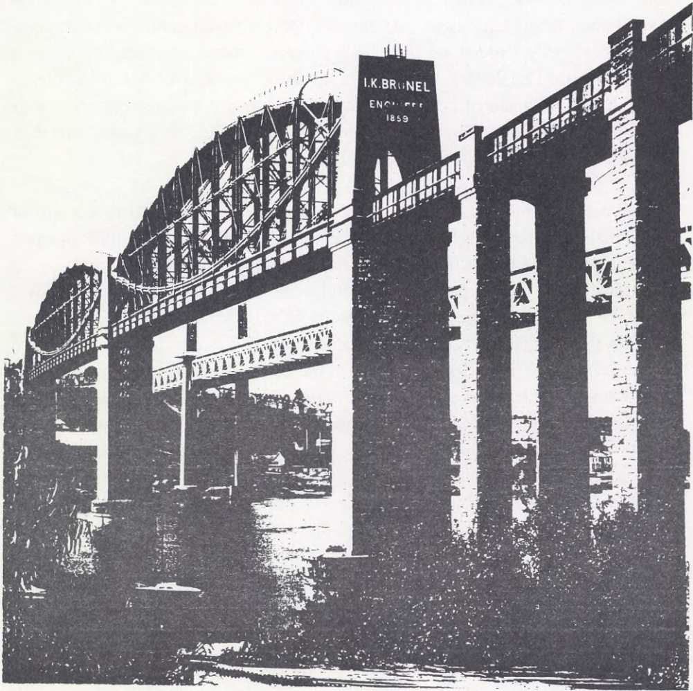
Saltash Bridge today.
