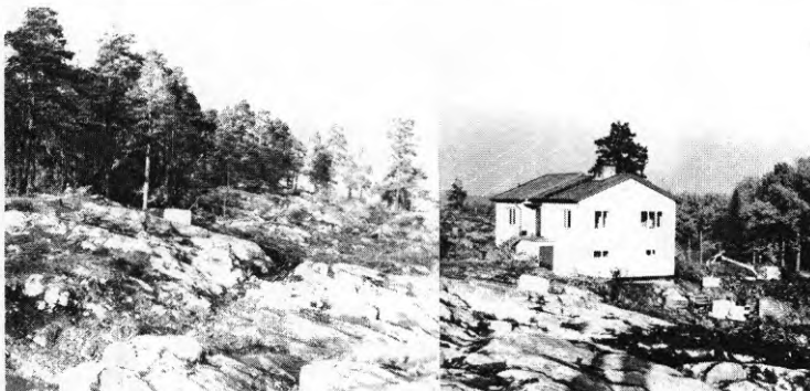
FIG. 1 Experimental house of light concrete, Älta outside Stockholm.
