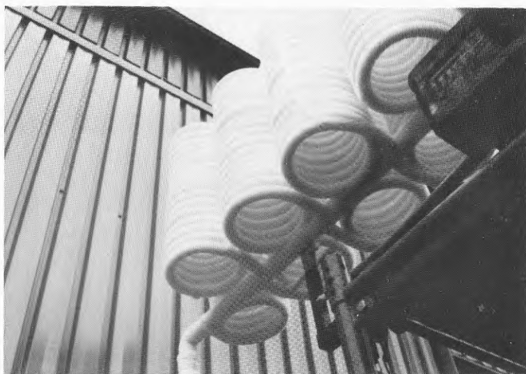
Fig 3.26 Helt igenfruset cylinderstaket
