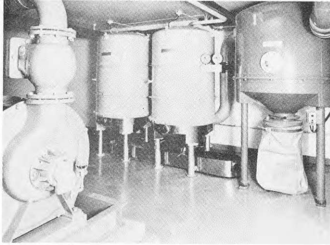
Fig 3:198 Apparatrum i centralt dammsugsystem
