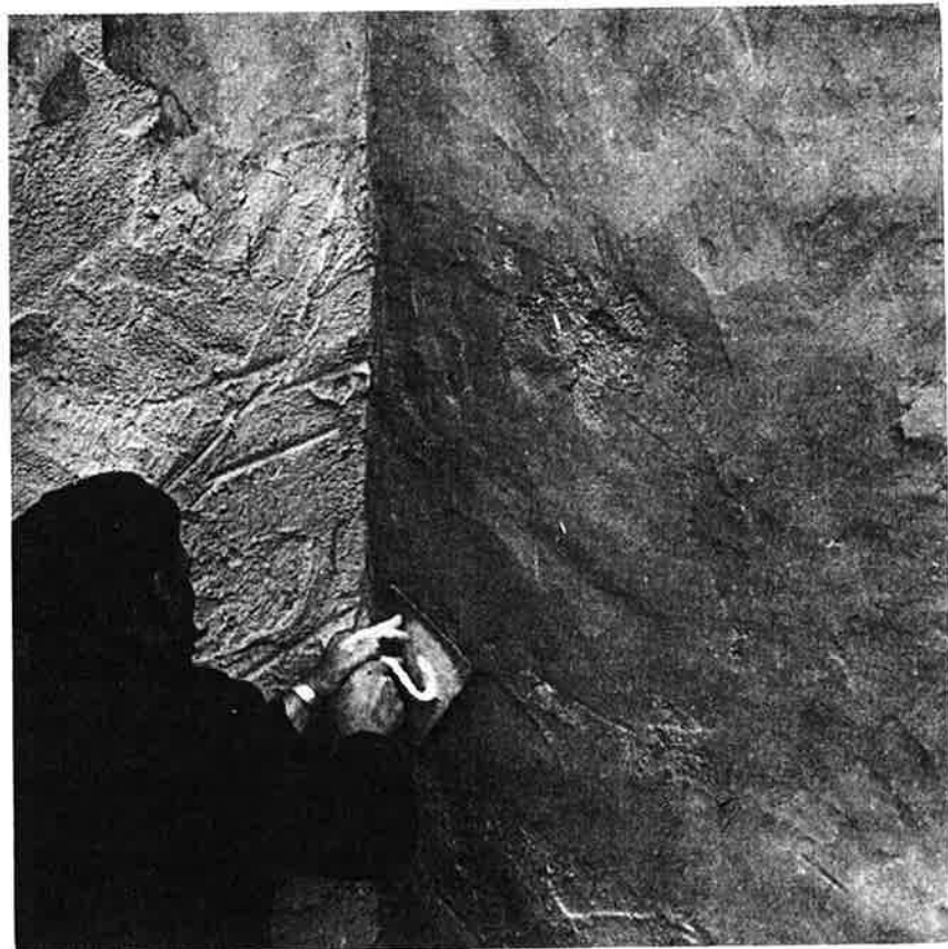
■ Fig. 25 and 26. In Gotland plastering- and rendering techniques, which can be identical with the medieval, have been used right up to modern times. Neither floete, spatula nor brush is used. After casting the mortar has been drawn off with the edge of the trowel (above, right). When the surface is dry, it is pressed and smoothed with the trowel till it is even (below, right). This technique is still used in the restoration of medieval plaster and gives it exactly the same appearance as this one
