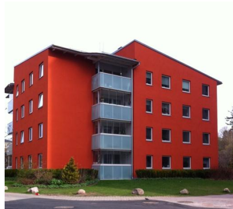
Figure 3 After the renovation of Katjas Gata 119
