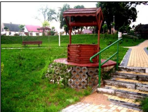
Fig. 6.12. Extreme ground level differences in the square of Denków; a cohesion failure that may be missed out by remote sensing. Photo: M. Dymitrow
