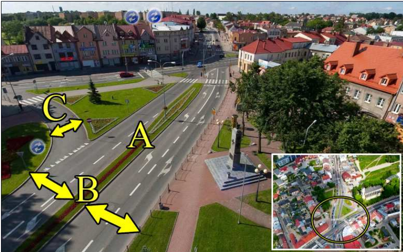
Fig. 6.8. Example of a street separator (A), dividing a four-lane road (B) that equals more than double the width of a standard-size road (C). Example from the market square in Grajewo.
