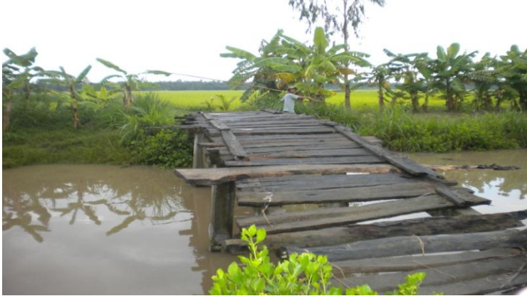
The wooden bridge
