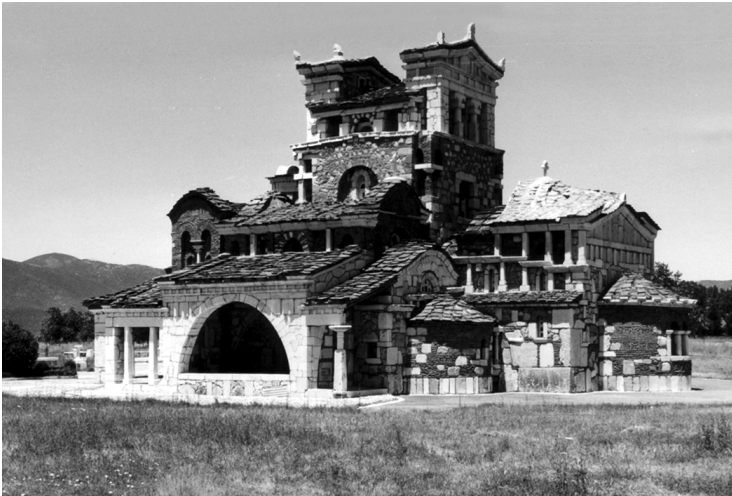
Fig. 6. Agia Fotini, Arcadia, Greece. One of the most unusual, modern churches in Greece: it is a mixture of Classical and Byzantine elements, influenced by Japanese pagodas, and was built in 1972 by an engineer from Tripoli.
